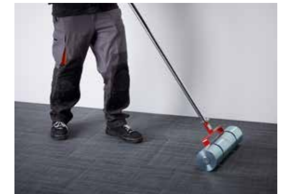
Smooth down the entire flooring area using the large, heavy roller.
