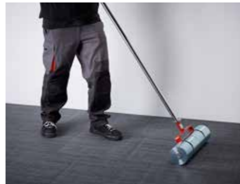
Smooth down the entire flooring area using the large, heavy roller.
